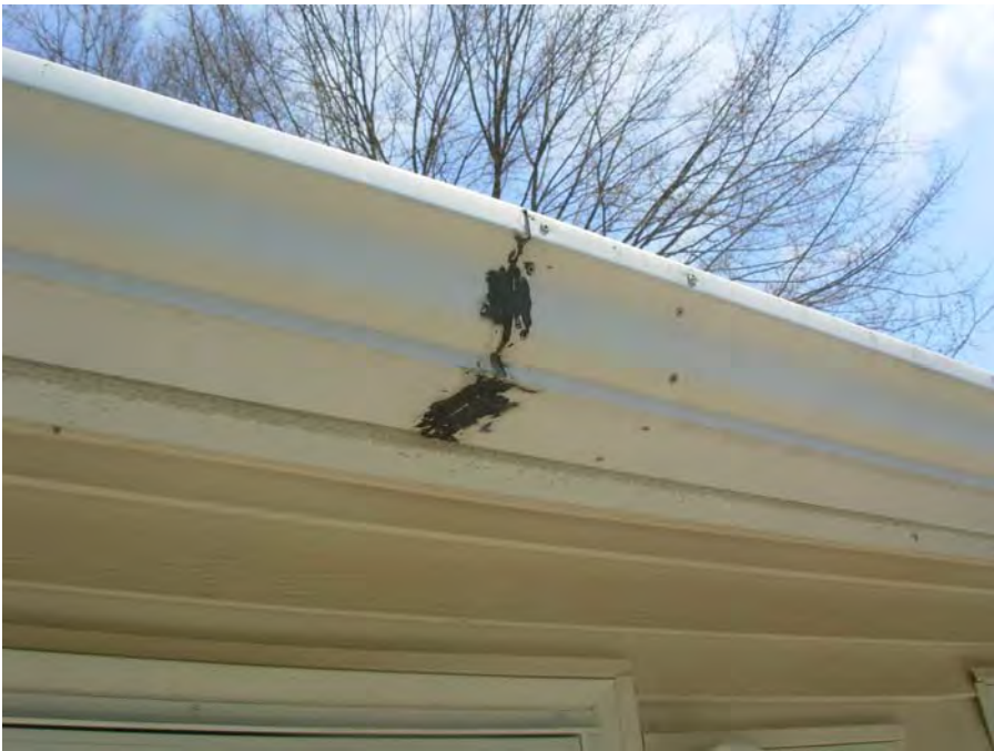
9. Gutter seam separation
