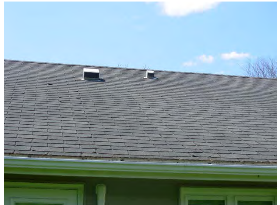
8. Lifting and curling of older roofing shingles
