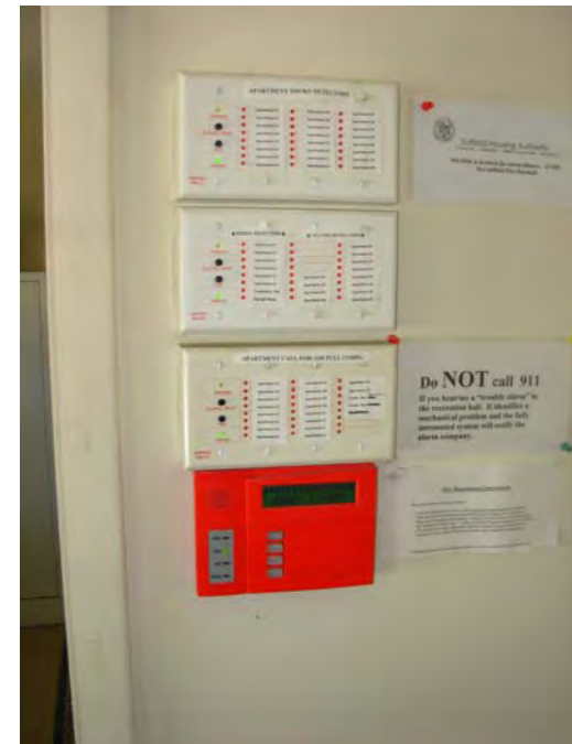
12. Fire detection - monitoring panel system
