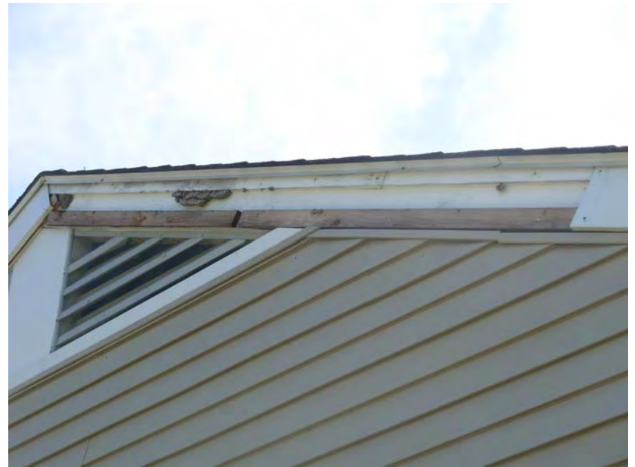
6. Spot rake board trim damage
