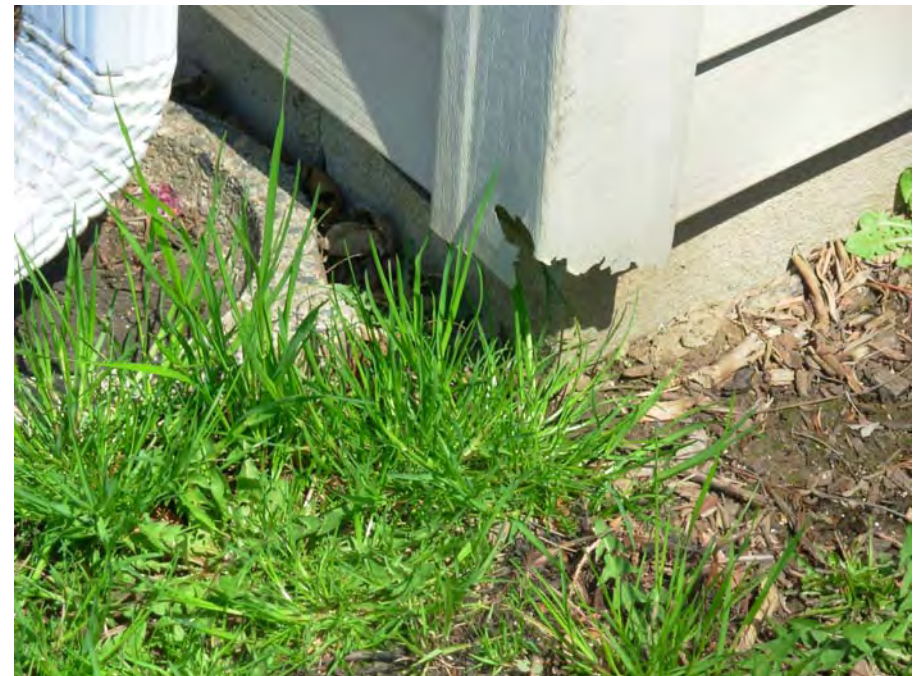
4. Spot vinyl siding damage
